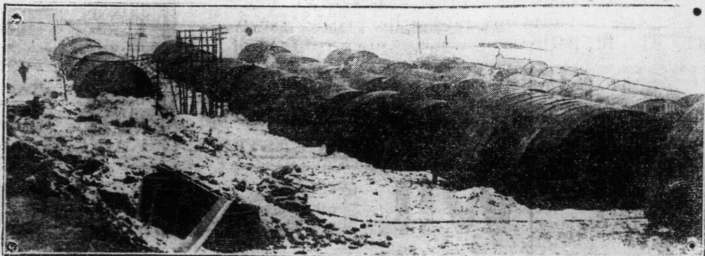
This is a British official photo taken on the western front, which shows a small village of "Nissen Huts," named after their inventor, a British officer. The houses are semi-circular in shape, the rounded portions sloping upward as a roof. Roof and sides are of corrugated iron, and the shelters are equipped with flooring, windows and a door. They are easily transported as the British gain ground.
