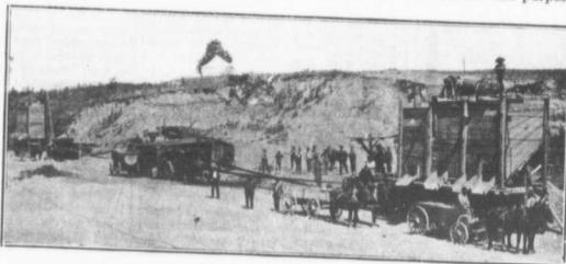
Stone Crushing in South Oxford—Coarse Gravel being used to make "Metal"
