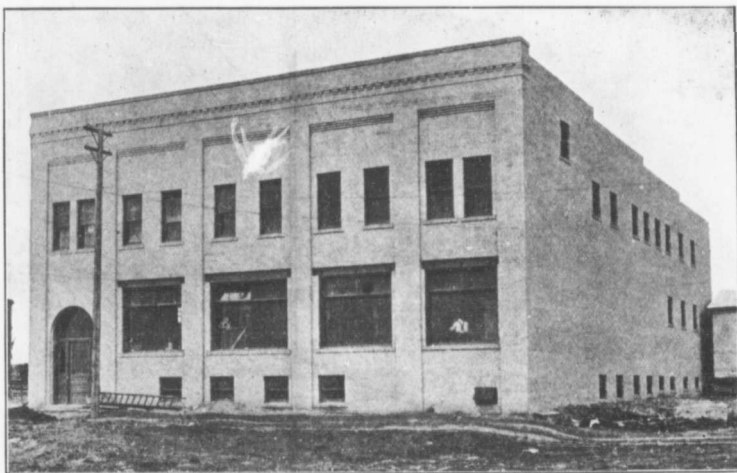
The Rex Fruit Company's new Warehouse in the Wholesale District, just completed, cost $28,000
