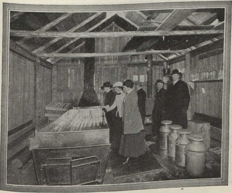
View of Inside of Sugar House, Maple Glen Reserve.
