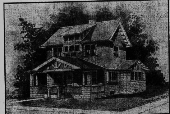
use cement in the construction of their homes we are illustrating in this week's issue a small cottage house, constructed of hollow cement blocks in the first story, with half-timbers and cement above the first story.
