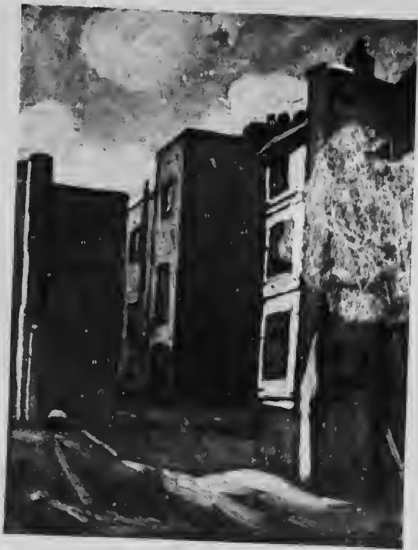
A TYPICAL LONDON DEMOLITION SCENE.
