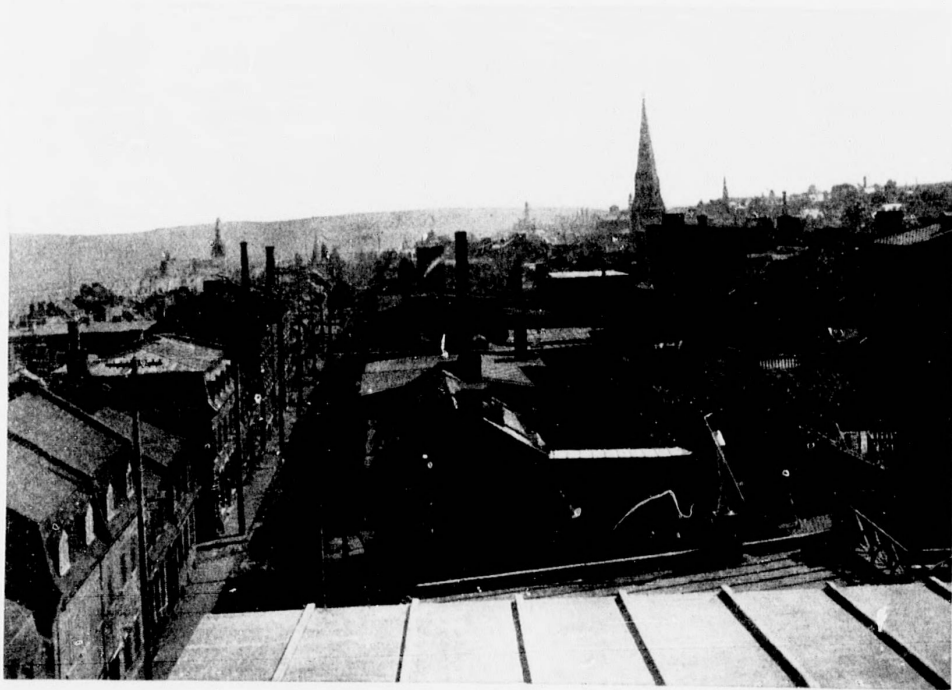
VIEW OF ST. JOHN STREET, EXTRA MURIS , LOOKING EAST.
