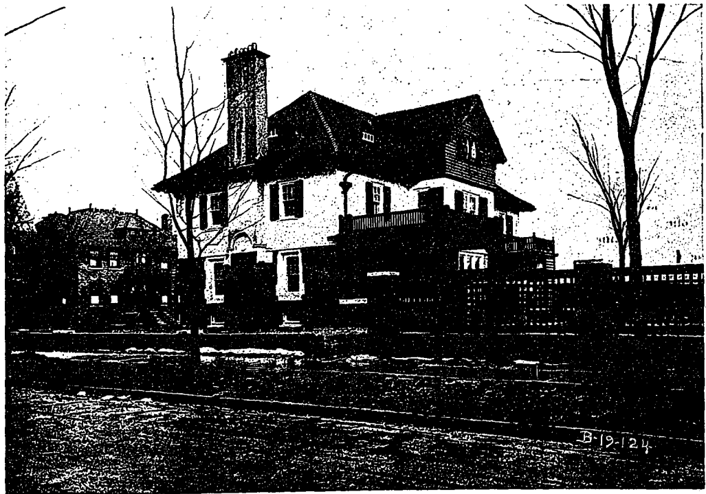
Front and side views, residence of Architect Albert Kahn, cor. Rowena and John's Streets, Detroit (Mich.). A thoroughly fireproof building that is not only commendable in design, but exceedingly interesting from a constructive standpoint. It is built in skeleton form, the structural frame being reinforced concrete, and the floors and walls a combination of reinforced concrete and hollow tile.
