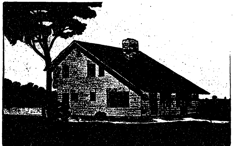
Rear view of Design No. 4 of suburban house, showing the broad sweep of roof. Note the slight projection in the shingled wall that forms a cap over each window or group of windows. This not only affords protection, but is a very interesting feature of the construction.
