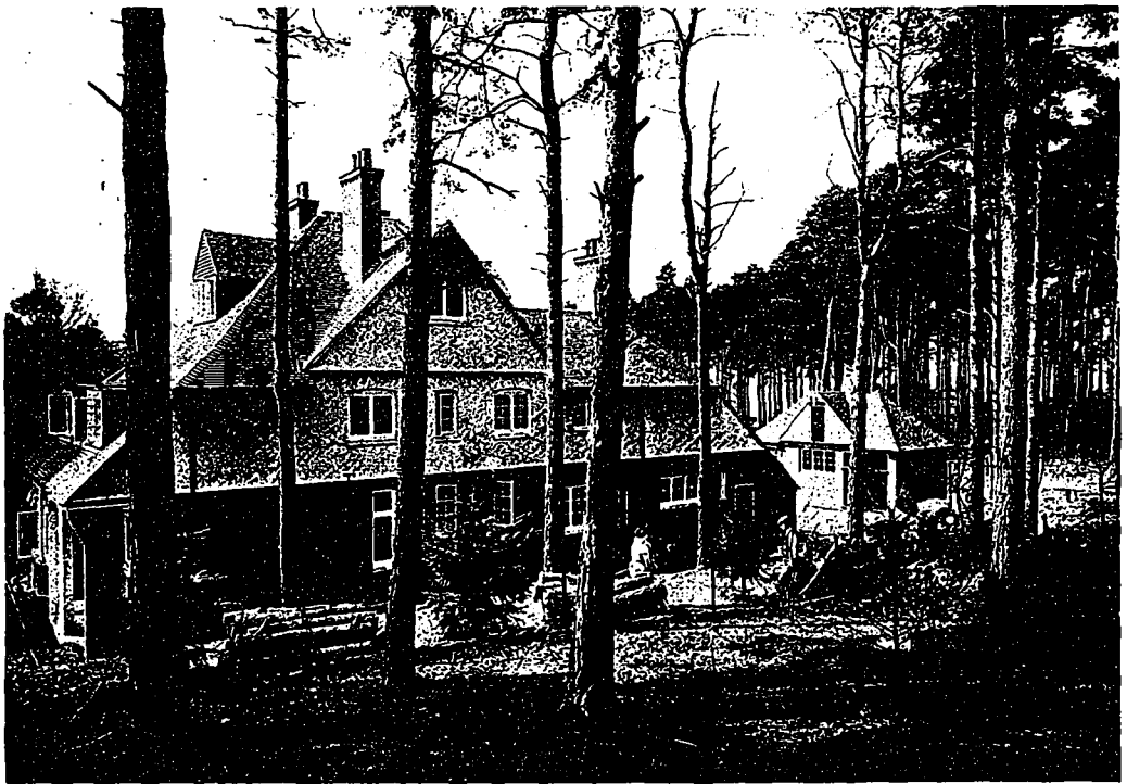
House at Camberley, as seen from the front and side. This home is built in the midst of a pine woods, a rather unusual site for an English house, but nevertheless one of a decidedly picturesque character. The building itself is a successful treatment carried out in red brick with rough-cast above, and a tile roof. One of its most striking features, and one which has greatly tended to enhance it from a viewpoint of design, is the interesting and architectural treatment of the windows and doorways. Mr. C. H. B. Quennell, Architect.
