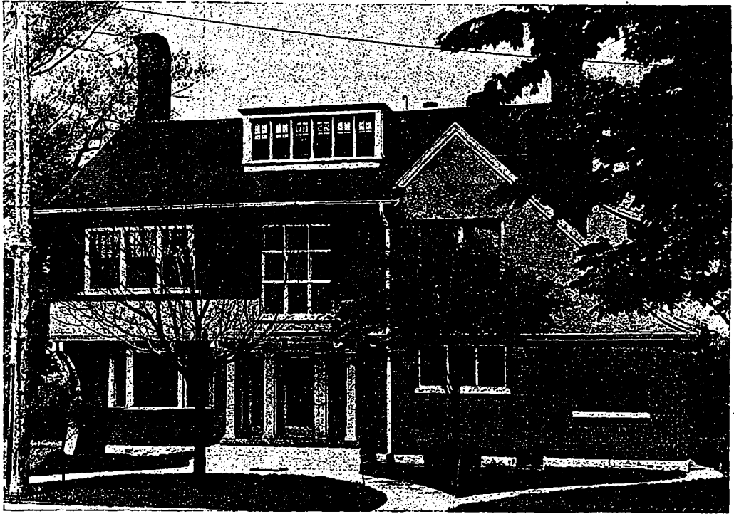
"Aitmover," home of J. McLenehan, Lamport Avenue, Toronto. A residence of noteworthy design, built of red brick for the first story, with cement stucco above. At the back it overlooks a deep ravine, and takes in a fine perspective of the picturesque bit of country stretching out toward the north beyond. Messrs. Wickson and Gregg, Architects.
