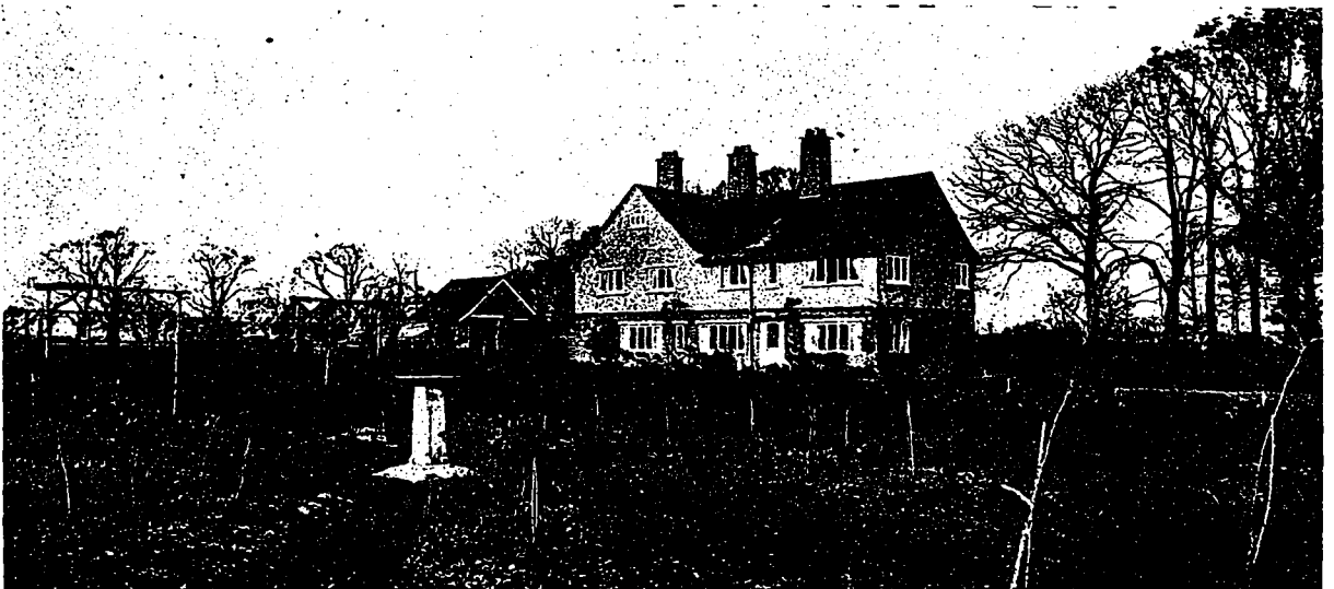
House at Biddenham, as viewed from the garden at the rear. The simple yet skillful manner in which this home is designed, has imparted to it a pronounced individual domestic character, that renders it unusually attractive. It is built of red brick, with the upper portion cement plastered, and a hand-made tile roof. Against this background, the white painted woodworks of the door and windows stand out in a pleasing contrast. Mr. C. E. Mallows, Architect.
