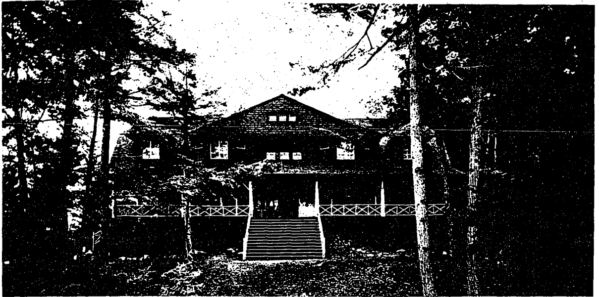
Cottage of Mr. Hepton, on Lake Joseph, Muskoka. A country home in rustic design, a type of building in which there is being developed an architecture characteristically Canadian. The outside clap-board and framing, left rough from the saw and stained a brown shade, together with the barked stripped cedar posts of the verandah, serve to make the general design of this residence strikingly effective. Messrs. Burke and Horwood, Architects.
