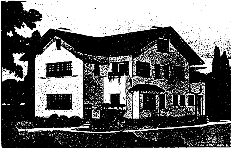
Design No. 1.—An eight-roomed cement house, suitable for a town, village or country. It is designed on simple lines, that harmonize with almost any surroundings. The walls are constructed of vitrified terra cotta blocks, directly upon which the plaster is applied, both outside and inside. The foundation is of field-stone, laid in black cement.
