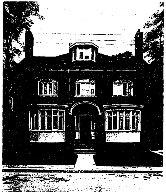
Home of R. L. Cowan, Rowanwood Avenue, Toronto. A clinker-brick residence of attractive design, which derives its chief charm from the variegated surface of its walls, and the simply decorative effect imparted by its doors and windows. Messrs. Chadwick and Beckett, Architects.
