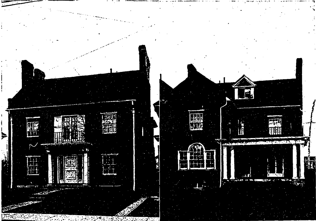
Front and rear views, Home of H. G. Kelly, Roxborough Street, Toronto. Aside from its pleasing architectural lines, there is a peculiar interest attached to the design of this house, in that the structure was especially planned and built around some very rare old Colonial furniture, so that the general exterior and interior scheme would be consistent in character. Messrs. Chadwick and Beckett, Architects.
