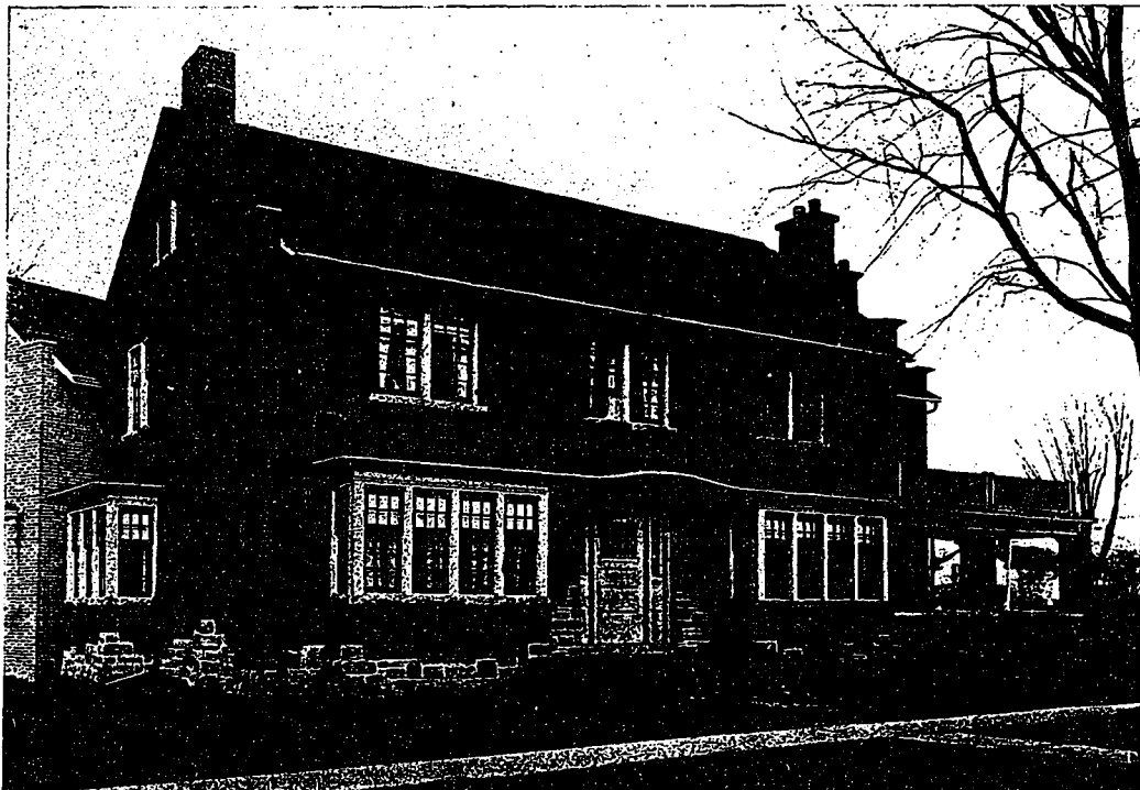
Rectory, St. Thomas' Church, St. Catharines, Ont. The directness of the general architectural lines, the simple treatment of the windows, together with the red brick walls, with their white joints and rustic base course, combine to give this house a strong homelike individuality. Mr. A. E. Nicholson, Architect.
