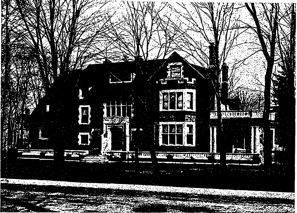
Residence of J. S. Ewart, K.C., Wilbrod Street, Ottawa. This building is designed with a modern English feeling, and simplicity in treatment has been observed. The terrace across the front prevents the building from having the high basement effect, which often spoils an otherwise pleasing structure. Mr. C. P. Meredith, Architect.
