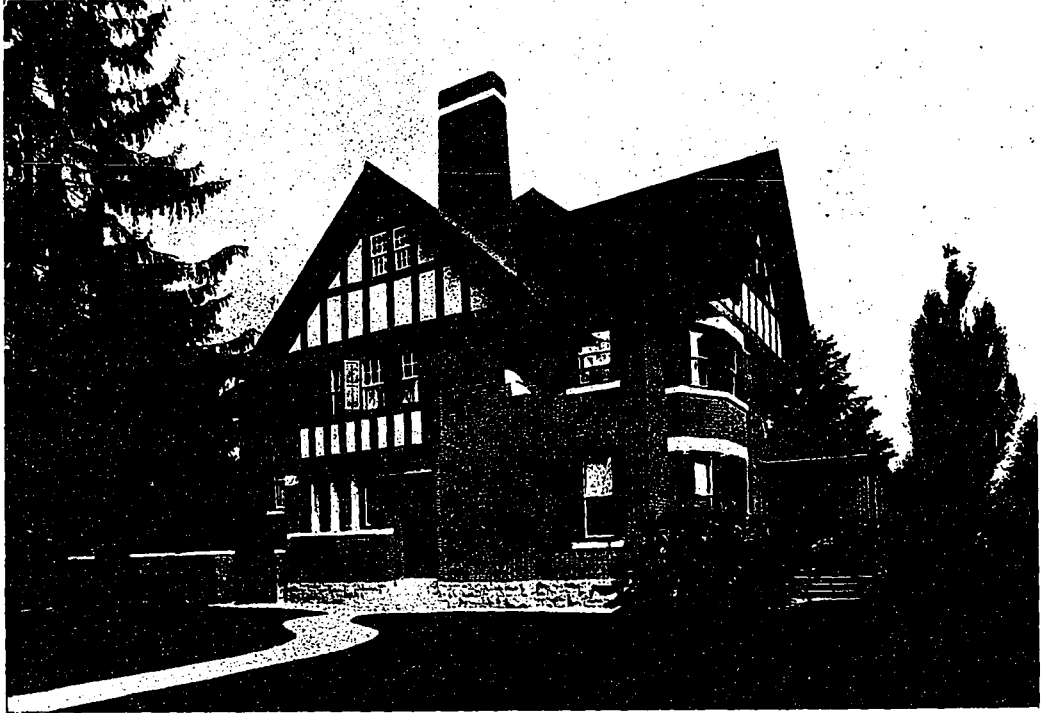
Residence of F. C. T. O'Hara, Wurtemberg Street, Ottawa. This house, which is situated on the high bank of the Rideau River, is built of common red brick, with white joints, limestone trimmings and half timbered gables. The large main chimney in the position it is placed suggests solitude and comfort, as well as adding interest to the whole scheme. Mr. C. P. Meredith, Architect.
