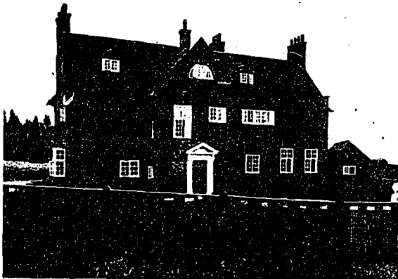
House at Elwell, looking towards the entrance. A simple, effective, brick building in which the only attempt at ornamentation is seen in the slightly emphasized quoins of the entrance bay and the arches above the windows. Mr. Guy Dawber, Architect.
