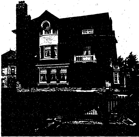
Residence of Edward Fisher, Crescent Road, Toronto. Messrs. Burke and Horwood, Architects.
