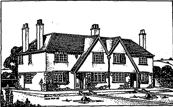
Pair of Houses at Glen-Cory, near Peterson-super-Ely, Glamorganshire. The design of this house has much to commend it in the way of a two-family dwelling. Its walls are built of rubble-stone with a roughcast exterior, the woodwork, with the exception of the oak porch timbers, being of red pine, and the roof of red tile. Messrs. Speir and Beavan, Architects.
