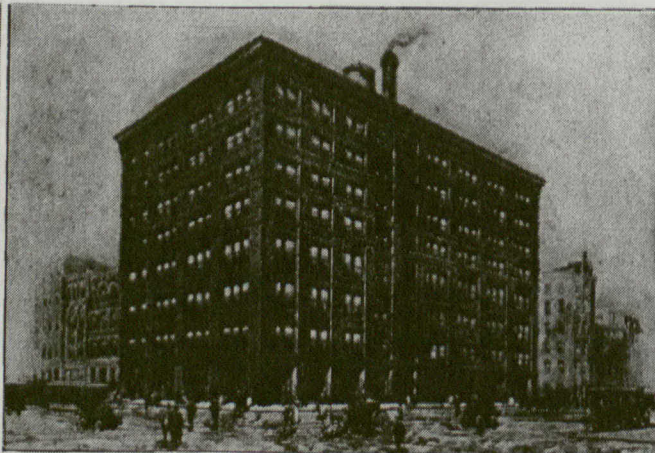
KETTERLINUS BUILDING FIRST REINFORCED CONCRETE SKYSCRAPER TO BE ERECTED IN PHILADELPHIA
