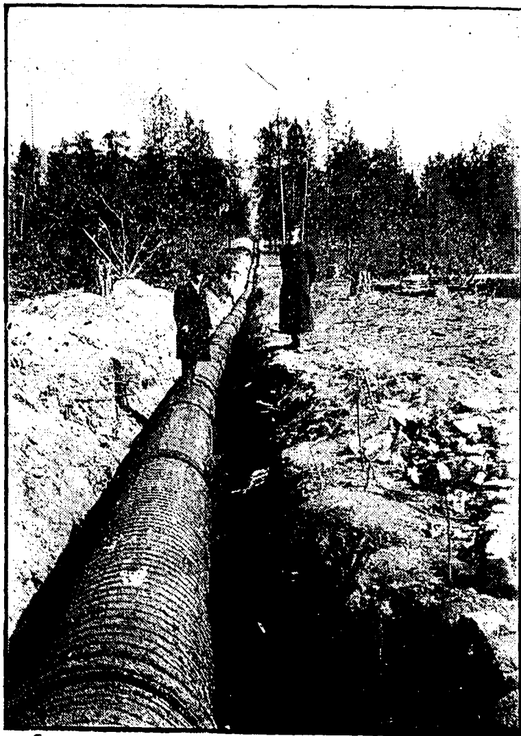
Part of Wooden Pipe System Installed at Okanagan Centre.
