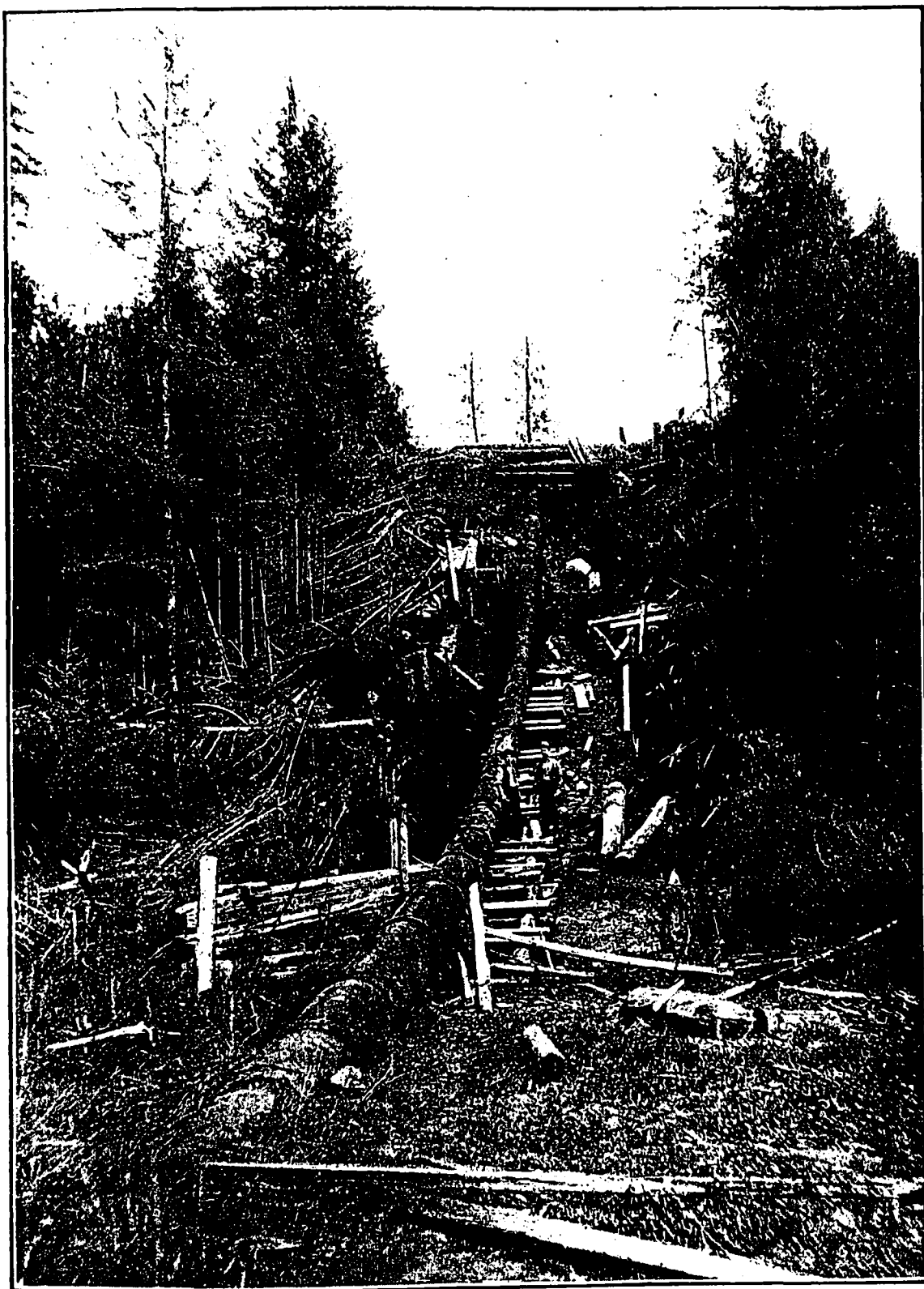
Pipe Line on Grey Canal near Vernon, B.C.
