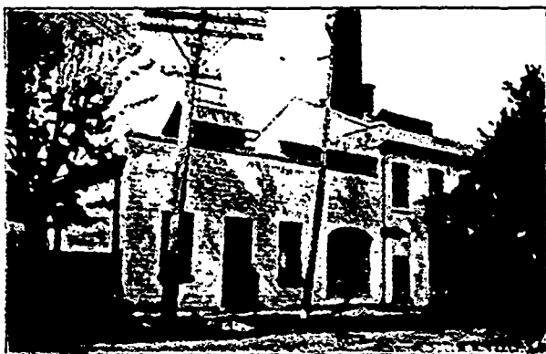
POWER HOUSE, KINGSTON LIGHT, HEAT & POWER CO.
