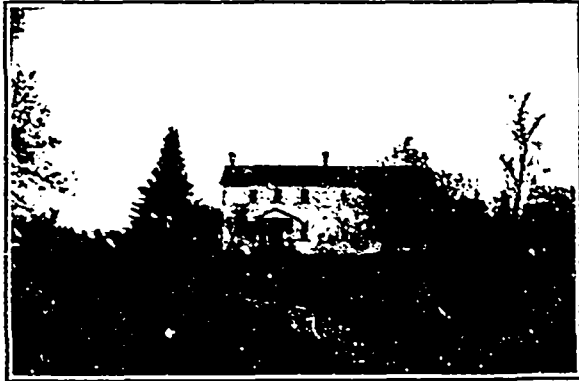
C. MISSEN'S RESIDENCE, CAMDEN
