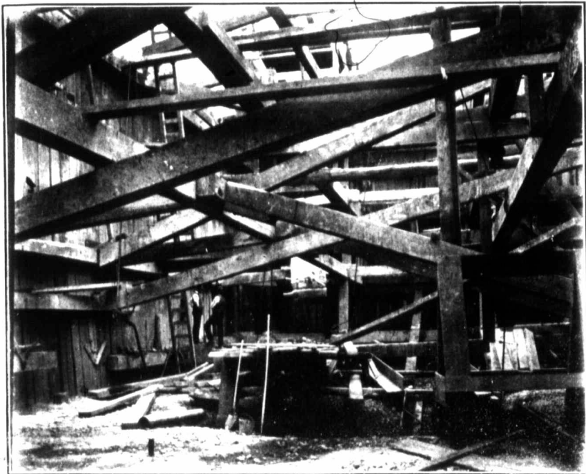
Showing temporary bracing required in foundation pit.
