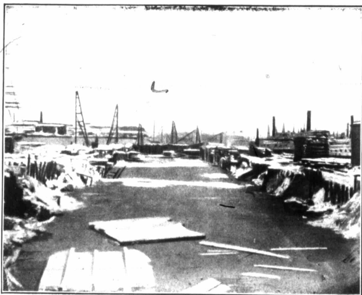
Driving piles from the Temporary Braces.
