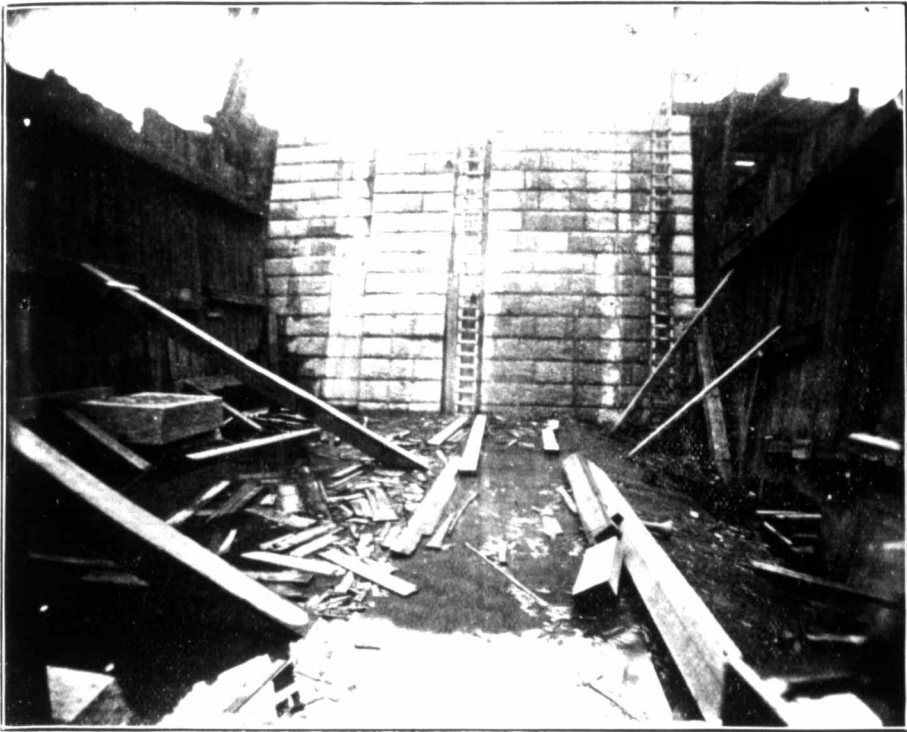
The Completed Abutment.
