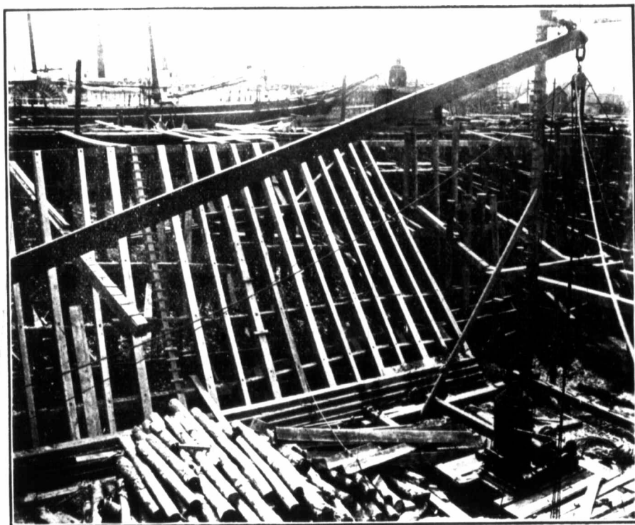
Shewing the side slope timbering.
