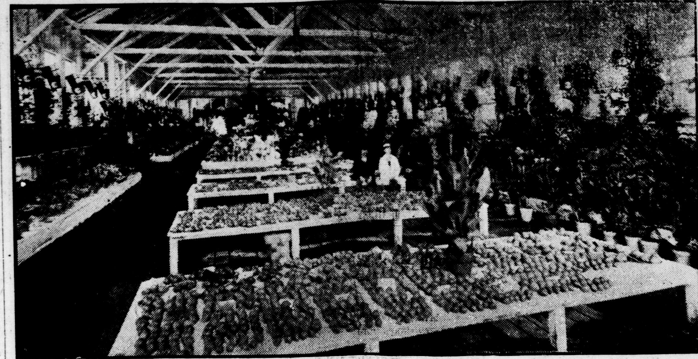
Interior View of the Horticultural Building.
