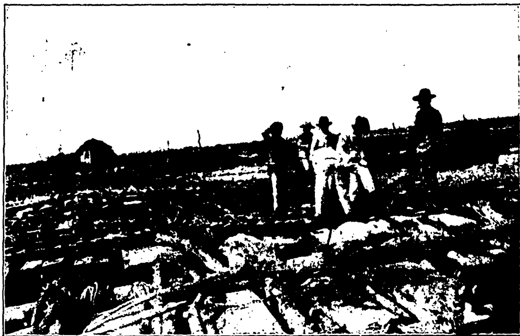
FIG. 1.—MEASURING LOGS IN RAFT ON TONDO BEACH, MANILA. THIS PICTURE SHOWS METHOD OF MAKING A RAFT BY TYING LOGS WITH BAMBOO STRIPS.
