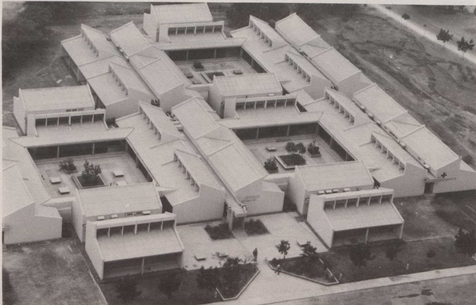
The Albert Royer hospital in Dakar, Senegal, is the winner of a prize for architectural excellence awarded by the Order of Quebec Architects.
