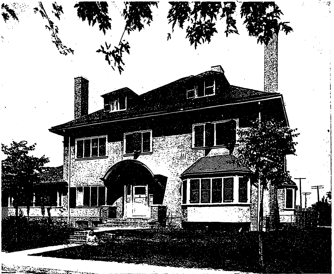
HOUSE NO. 2—ANOTHER EXCELLENT EXAMPLE OF DOMESTIC ARCHITECTURE, IN WHICH THE ARTISTIC APPLICATION OF CEMENT STUCCO ON BRICK IS FAIRLY DEMONSTRATED. ONE OF THE FEATURES OF THIS HOUSE IS THE DEEP VERANDAH WHICH IS REACHED THROUGH THE LIVING ROOM LOCATED OFF THE RECEPTION HALL. EDEN SMITH AND SON, ARCHITECTS.
