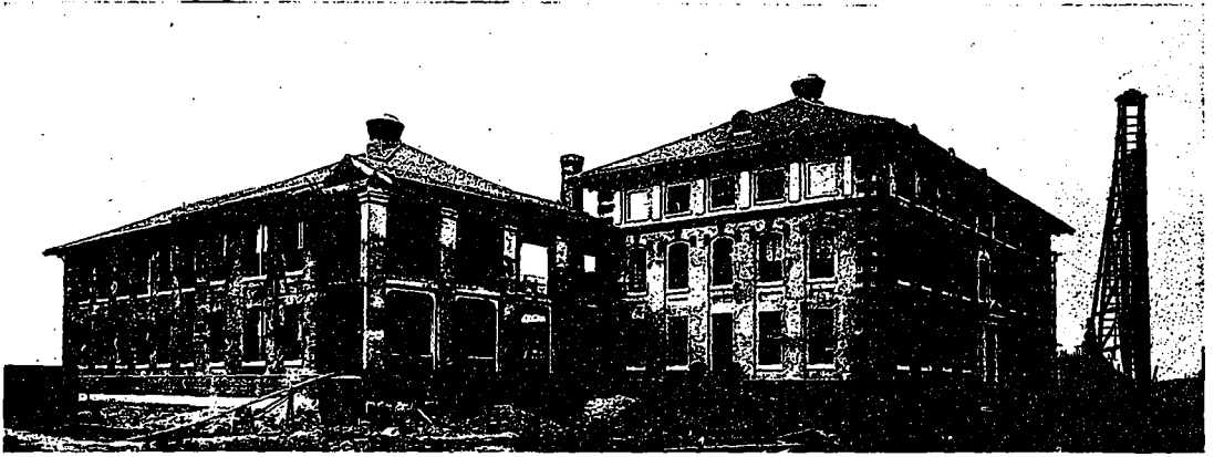
VIEW SHOWING TWO OF THE NEW HOSPITALS FOR CONTAGIOUS DISEASES, U. S. IMMIGRANT STATION, ELLIS ISLAND NO. 3, EACH OF WHICH RESTS ON CONCRETE PILES. A FEATURE OF THE EXTERIORS OF THESE BUILDINGS IS THE MANNER IN WHICH THE TERRA COTTA TILE HAS BEEN USED FOR TRIMMINGS AND ROOF TO RELIEVE THE DEAD GRAY COLOR OF THE CONCRETE WALLS. A CONCRETE PILE DRIVER MAY BE SEEN AT THE RIGHT.
