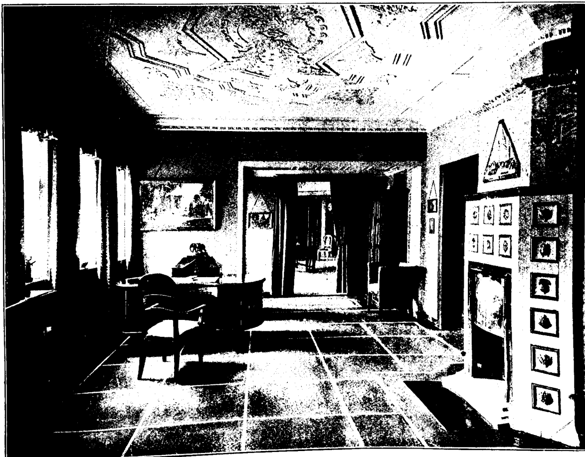
Showing Doloment Flooring as Used in Business Office.
