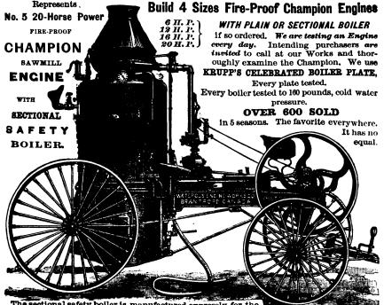
sectional safety boiler is manufactured expressly for the "North West" trade. This boiler is so arranged that it is readily taken apart in sections enabling purchasers to clean thoroughly every part of it and prevent burning out. We know from experience this is absolutely necessary with the alkaline waters of the great Western prairies. Largely used by the Pacific Railway Company and all the large Colo-
