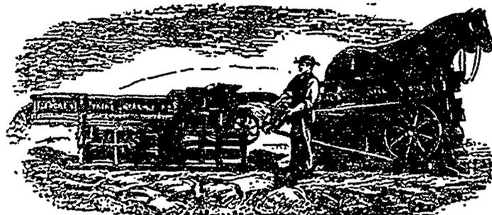
The thrashing machine represented in the above engraving is our vibrating machine. It has a run of 24 inches long with teeth in steel guaranteed so that they can bend without breaking as the norway.
