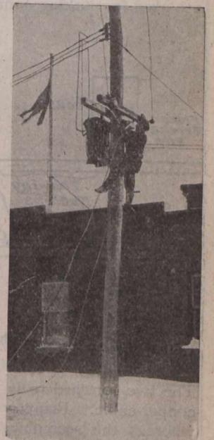
Fig. No. 2.—Connecting the Primary Leads to the 2,200-Volt Circuit
