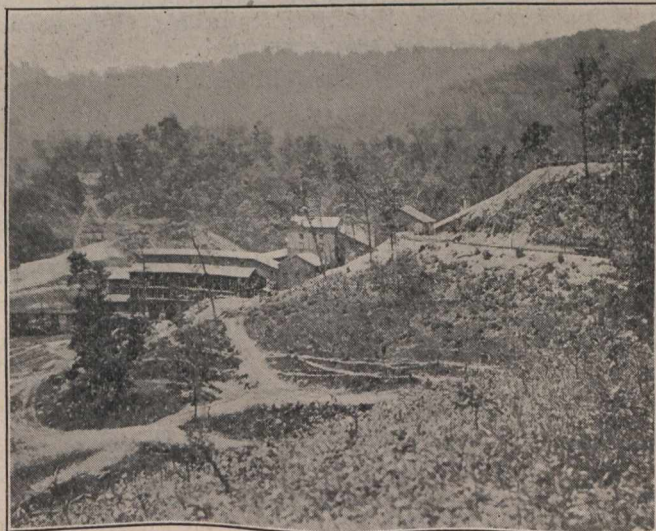
Coal Tippie, showing elevation at which coal is dumped.
