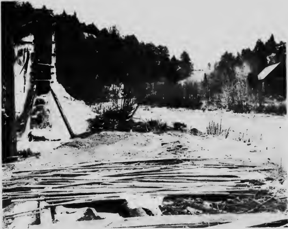
Dam, Old Mill on the Left and Electric Light Plant on the Right. Bear River, N.S.
