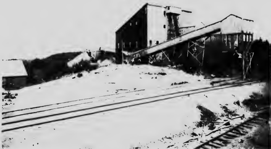
Iron Ore Separator. Operated Electrically with Power from Nictaux Falls, Nova Scotia.
