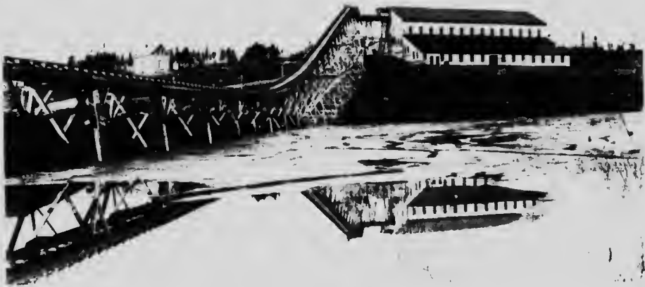
Gold Mine Building and Tramway, Isaac Harbour, Nova Scotia. Operated Electrically.
