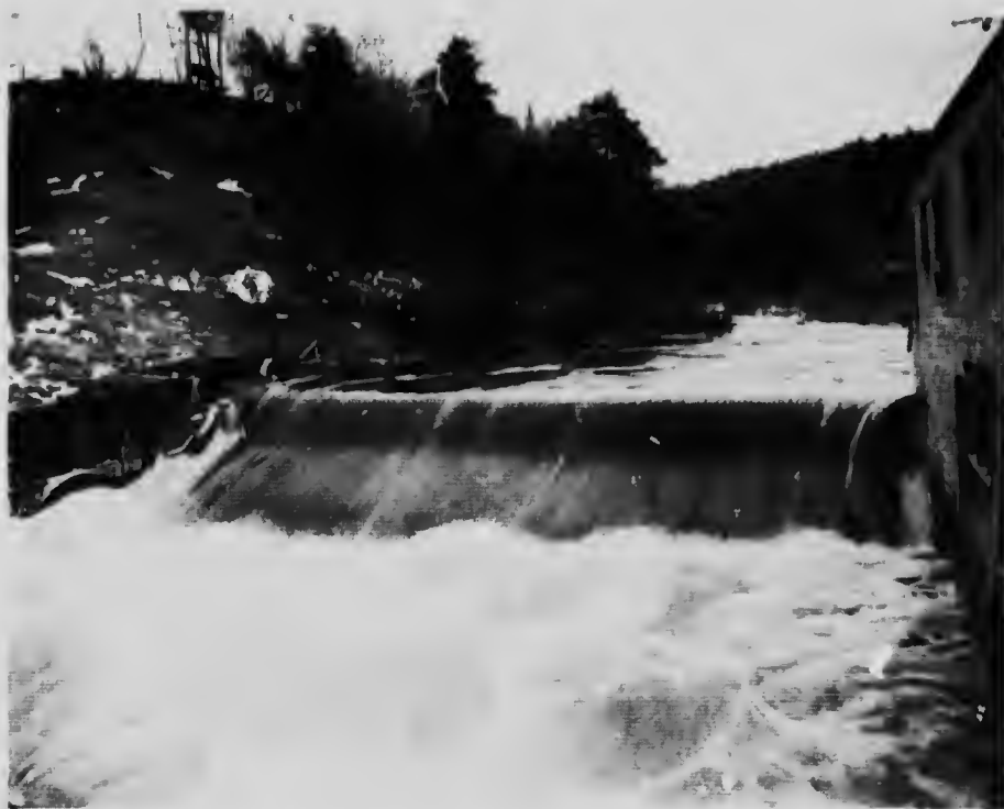
East Branch, Bear River, N.S., at Head of Tide-water. Granite Works on Right.
