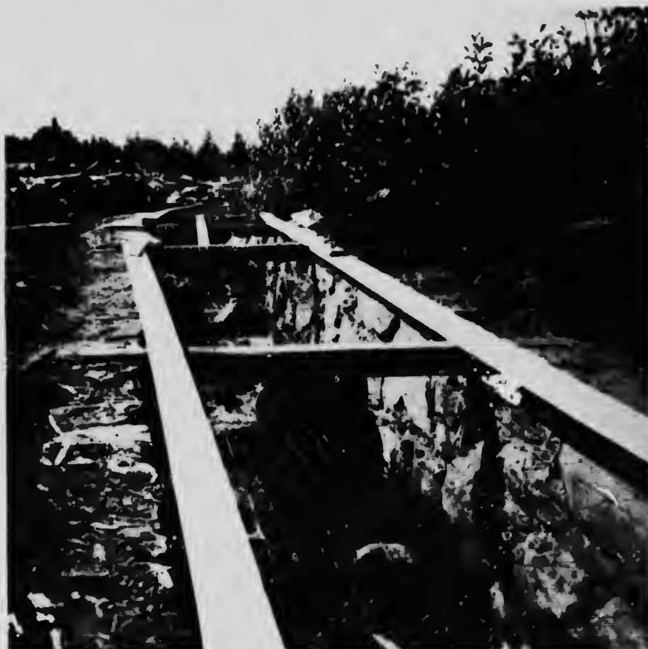
Fish Ladder. Lower Pulp Mill Dam, Mersey River, Nova Scotia.
