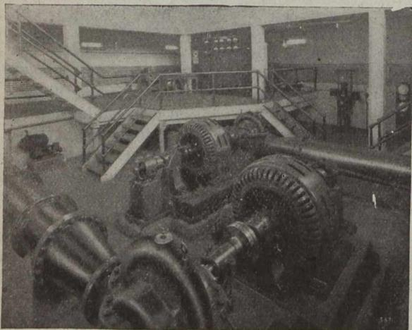
Motor-Driven Centrifugal Pumps, 5,000 Gal. Per Min. Each Against 171 Ft.
