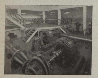
Motor-Driven Centrifugal Pumps, 5,000 Gal. Per Min. Each Against 171 Ft.
