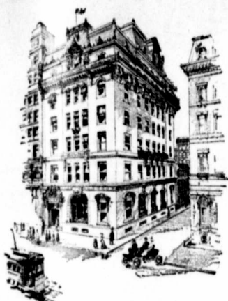
CANADIAN BRANCH LONDON & LANCASHIRE LIFE HEAD OFFICE BUILDING, MONTREAL B. HAL. BROWN, GENERAL MANAGER.
