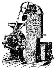
As shown, are now fitted with a Shaking Screen to take out all Straws, Stones, Nails, Cyl. Teeth, etc.
