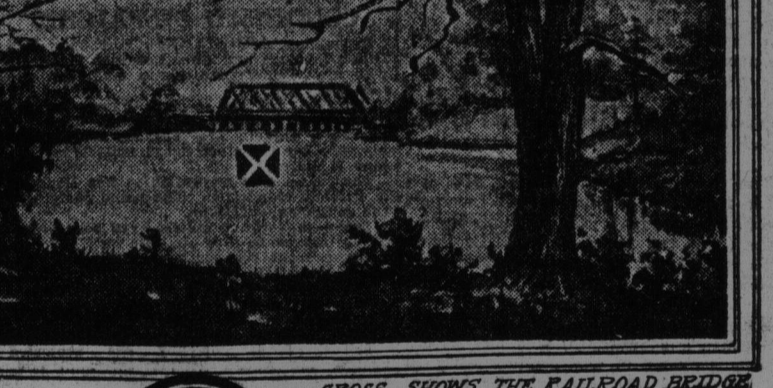
CROSS SHOWS THE RAILROAD BRIDGE WHERE PIERSON WAS KILLED.
