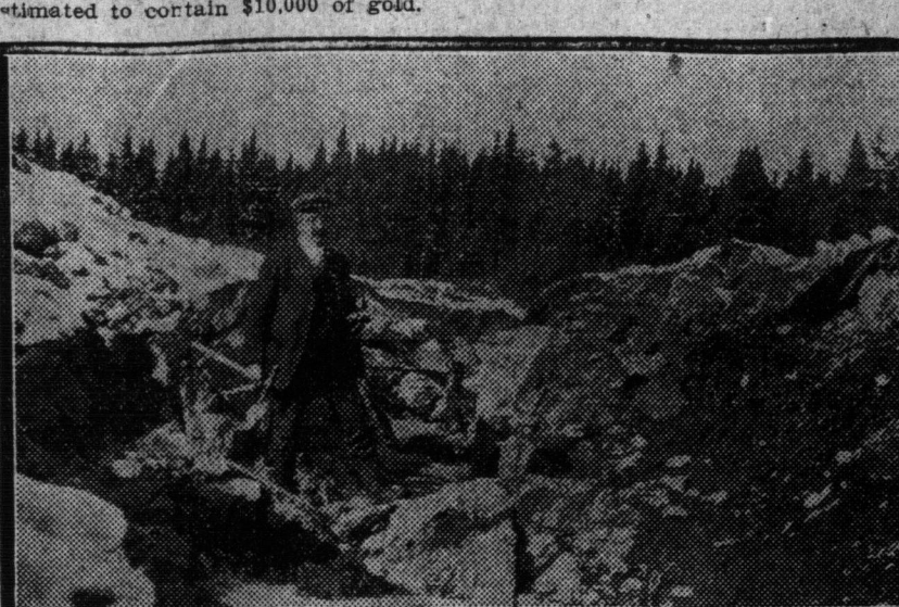
The open cut from which the above ore was sucked. Work is being continued on this chute.
