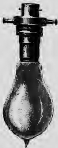
FIG. 88.—LAMP SOCKET FITTING WITH CONNECTIONS FOR CHARGING SECONDARY CELLS FROM THE MAINS THROUGH THE LAMP.
