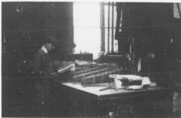
Apprentice at work on marking off table, Canadian Pacific Angus Shops, Montreal.
