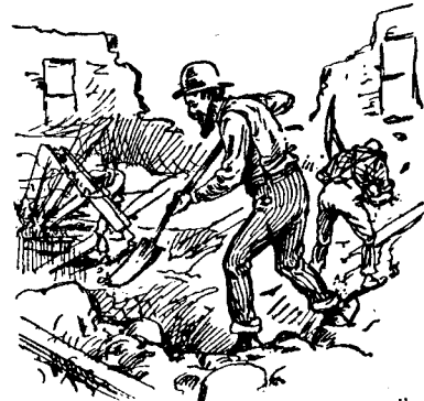
"I was helping dig out the cellar."
