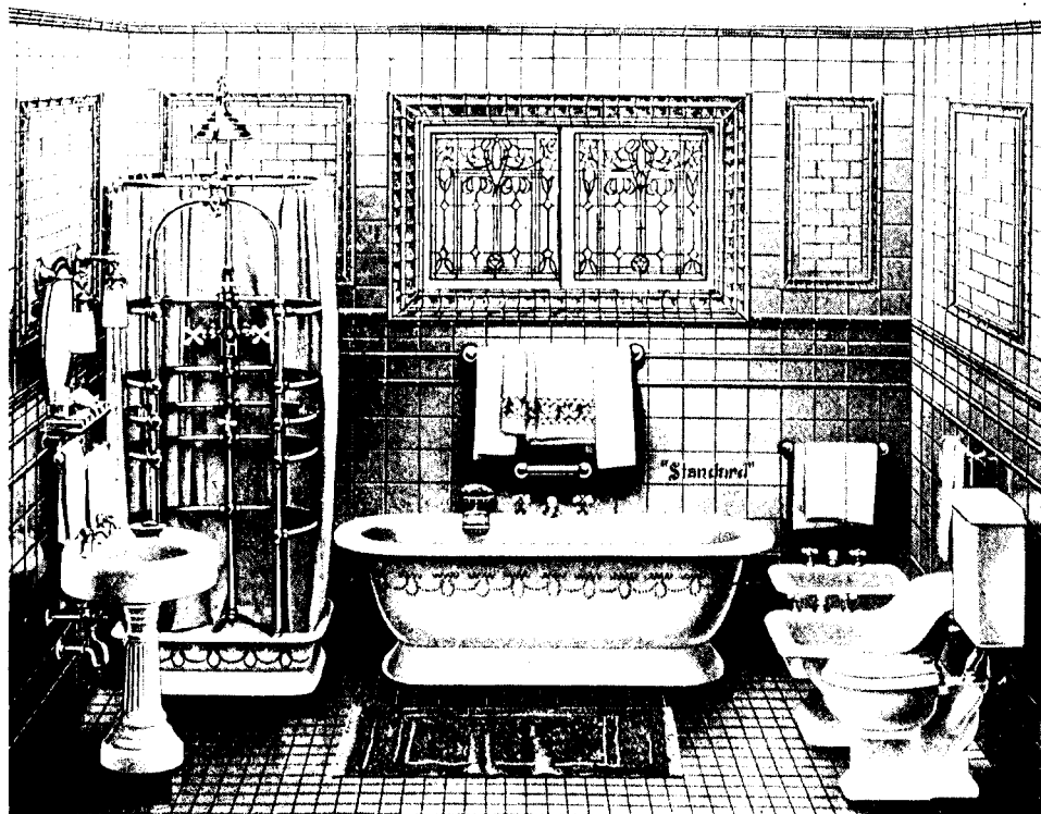
“Standard Sanitary” Bathroom of Queen Victoria of Spain.
