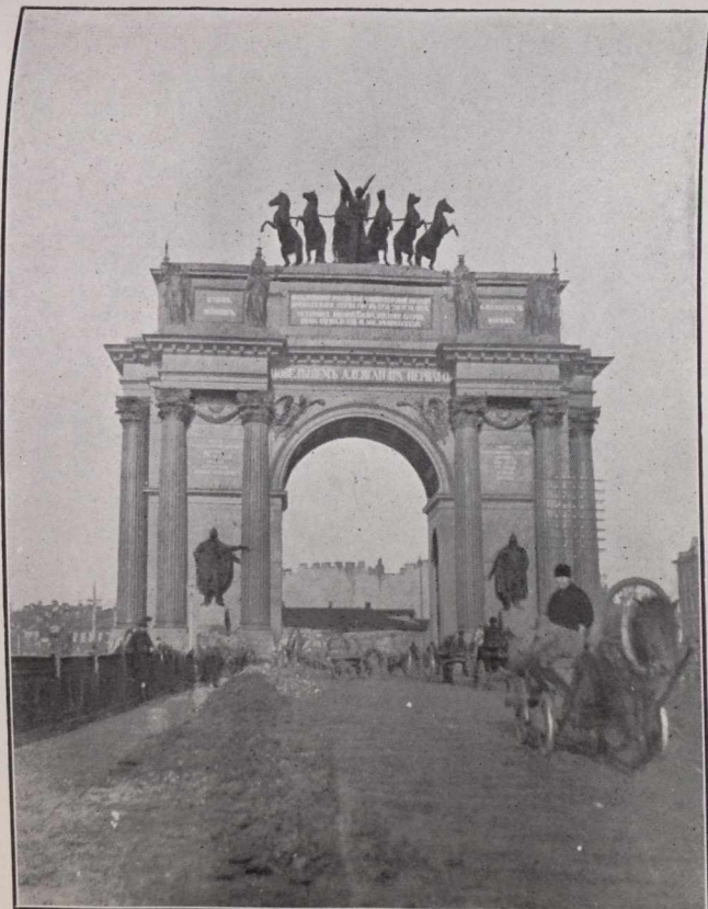
" Near the Putiloff Iron Works is a fine stone archway, which had been newly painted and gilded to conceal all traces of the terrible conflict which waged about it on the 22nd January. "
