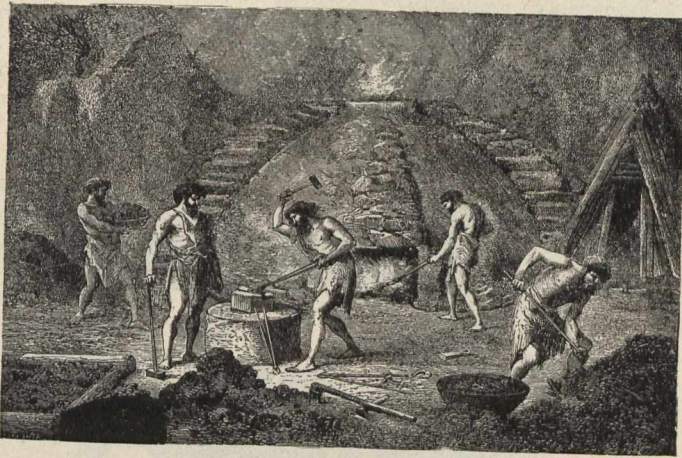
Fig. 3—Primitive Furnace for Smelting Iron.
