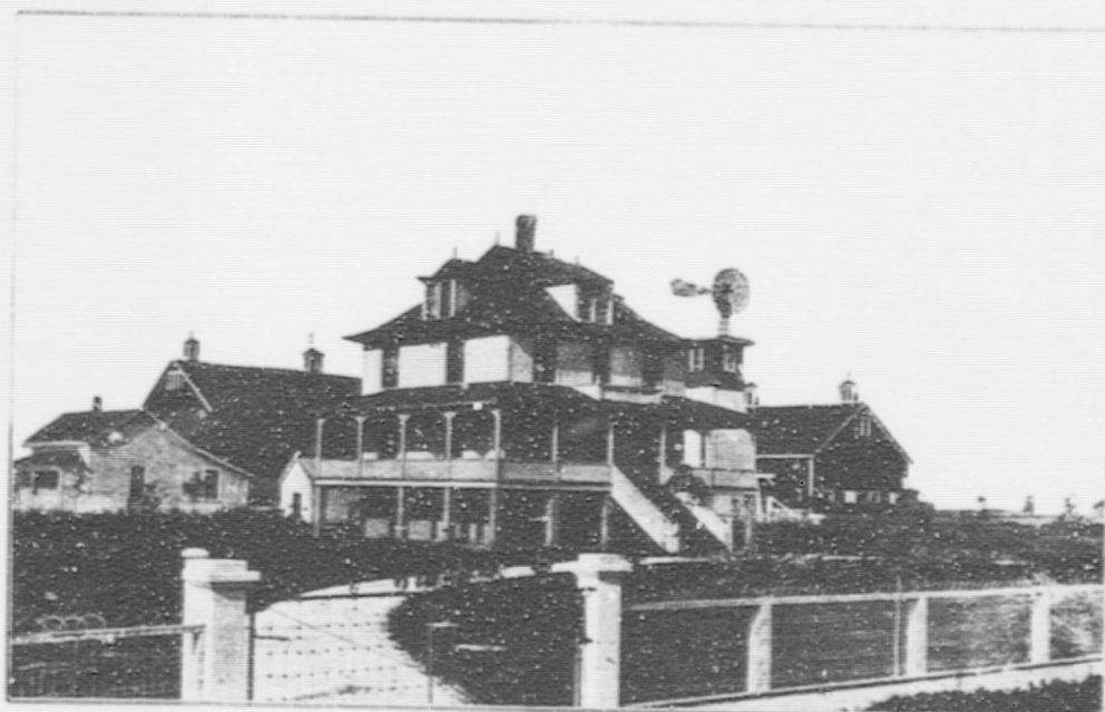
Manager's Residence on the 6000-Acre Burns Ranch
