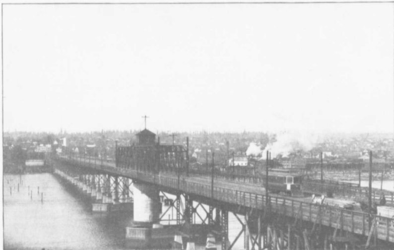
High level steel bridge, Granville Street.
