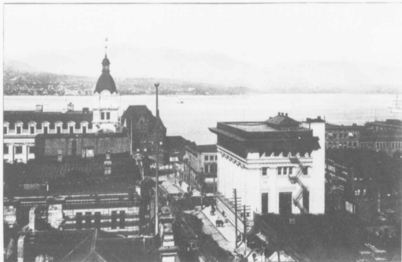
Corner of Granville and Hastings Streets, North Vancouver in the distance.
