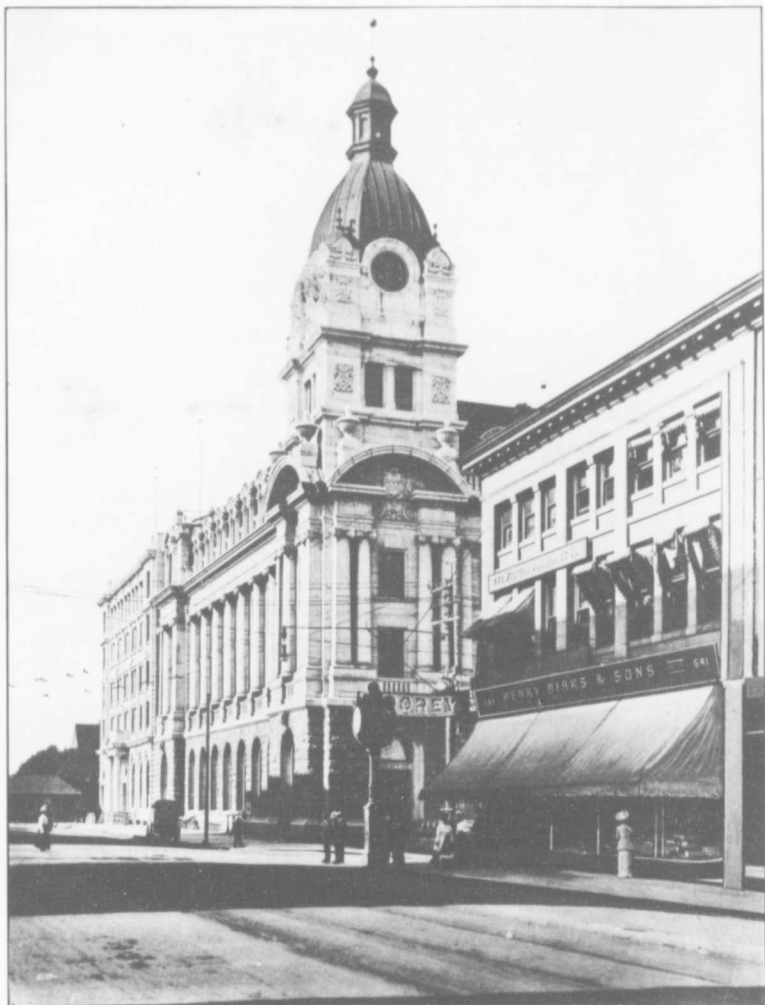
The Post Office, corner Hastings and Grinville Streets.
