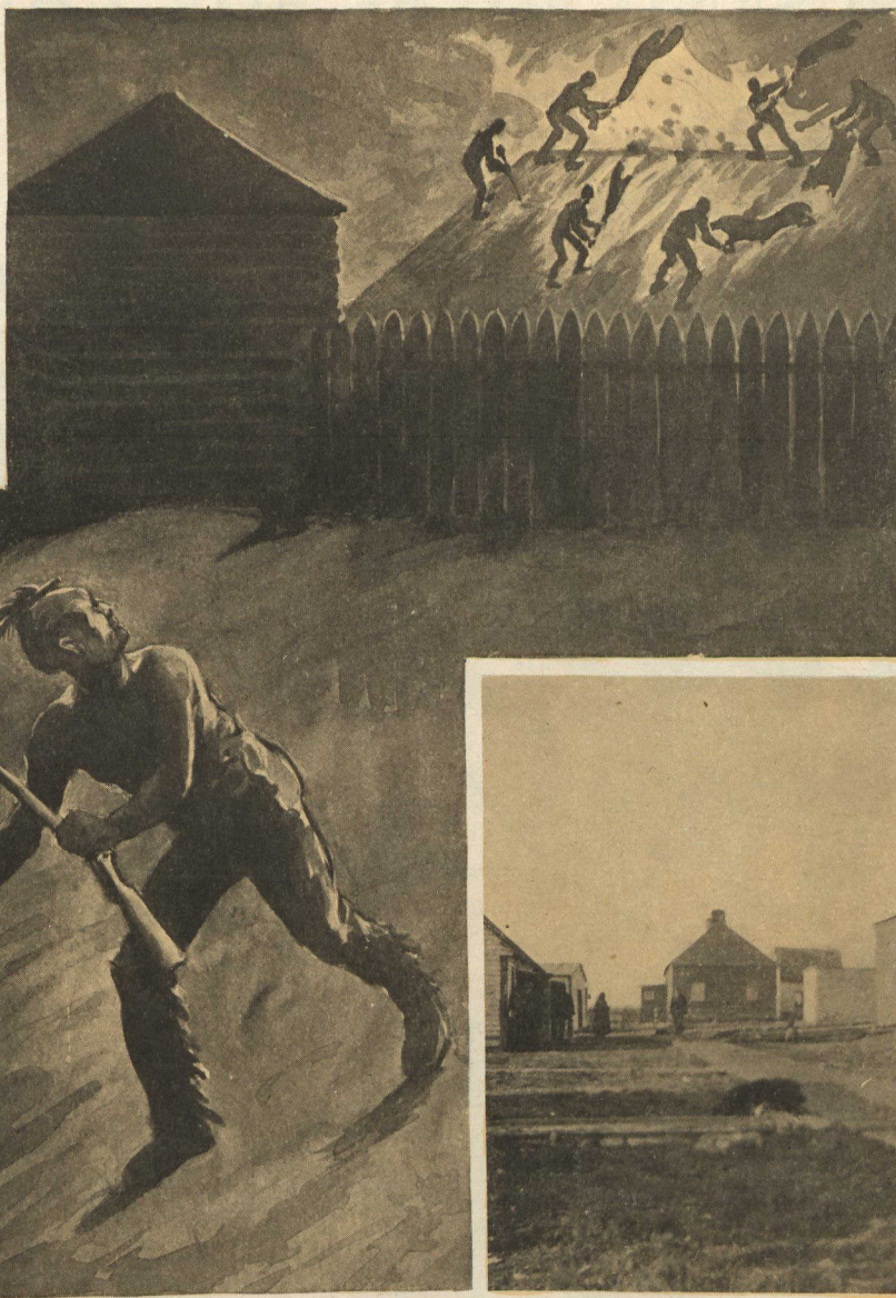
"Flogging out the fires in full view of the camp above and the fire-fiends below."
