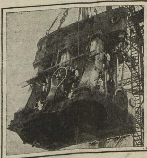
Hoisting 80 tons of Engines from old ship.
