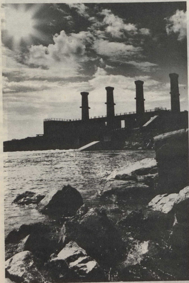
The lobster control structure, kingpin of the Churchill Falls hydro-electric power development's huge reservoir system, central Labrador, is one of six concrete structures that will regulate and control the flow of water to the 7-million horsepower underground power-house.
