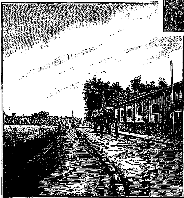
A CORNER OF THE BARN, MENIER ESTATE.
