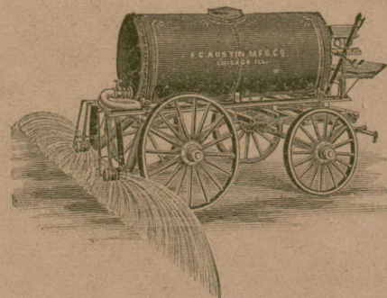
AUSTIN STEEL STREET SPRINKLER
