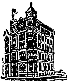
HEAD OFFICE BUILDING, MONTREAL.
