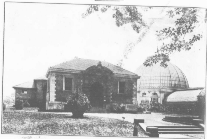
DETROIT.—AQUARIUM AND HORTICULTURAL BUILDING ON BELLE ISLE.
