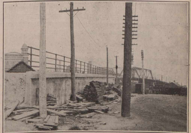
Fig. 4. View Showing Retaining Wall and Approach to Viaduct.
