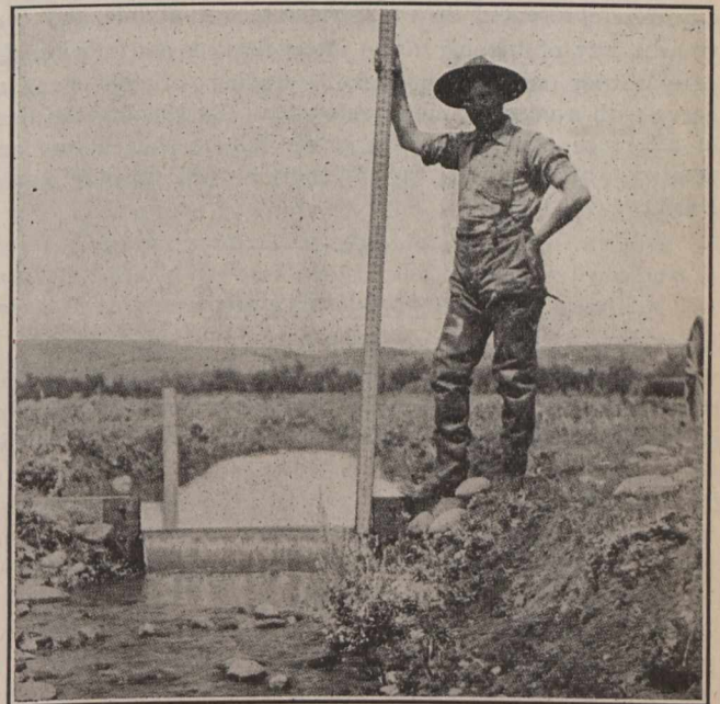
Thirty-Six-Inch Sharp Crested Rectangular Weir Used on Small Streams.
