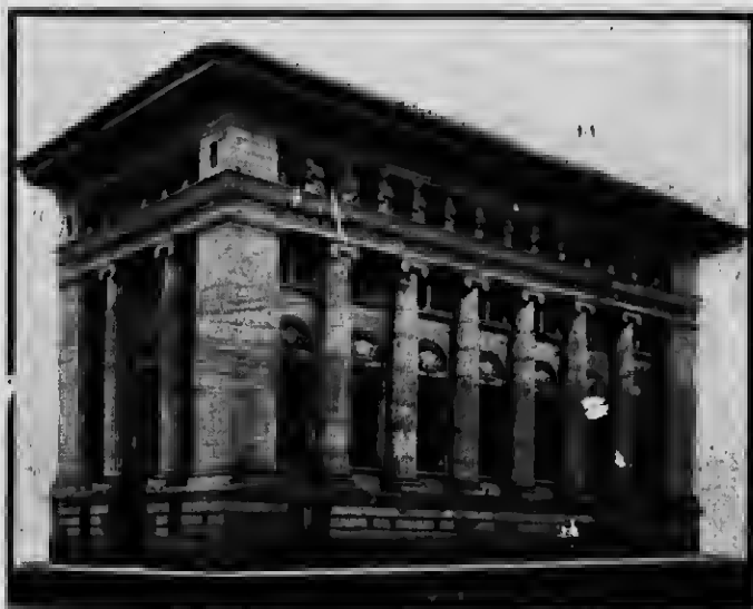
ONE OF VANCOUVER'S BANK BUILDINGS
