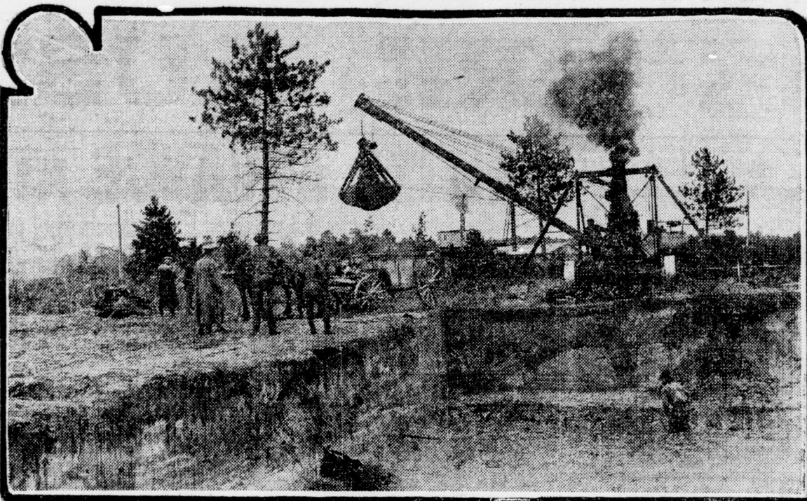
Portable steam digger working on septic tank that will treat all sewage at Camp Borden.
