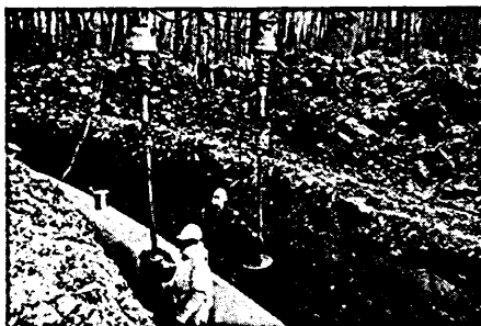
Installation of pipeline anchors.
