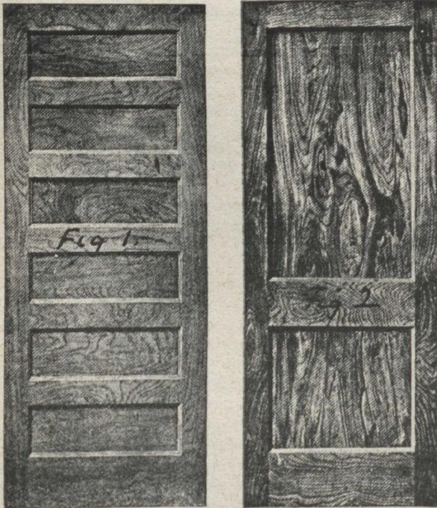
The type of door shown in Fig. 2 furnishes an excellent opportunity to show off good veneer work, especially in panels. It consists of two large panels, the top one full width running practically two-thirds of the length, and the
