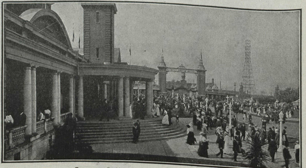
Government Building and Western Entrance to the Grounds
