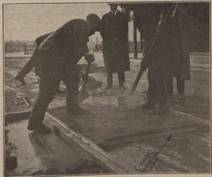
SQUEEGEING PITCH INTO JOINTS
